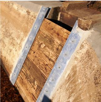
The brackets holding the spillway boards were rusted and the engineer suggested they be replace after the project was otherwise completed. The before and after pictures are shown above. A closer view looking down the brackets showing the thickness is below.
