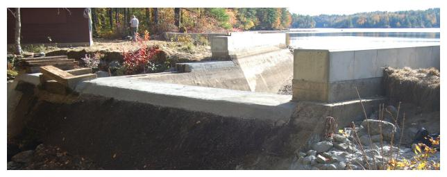
The increased abutment heights can be seen on both sides of the dam in the above picture, they are the lighter color. They were raises about 14 inches. The rebar can be seen in the picture below. The vertical pins with the orange caps (put on only for safety, and later removed) are drilled into the existing abutments and take the sheer force, the U-shaped pieces are to hold the poured cement together under stress.
