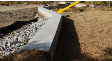
The abutments were extended on both sides from where the yellow arrows indicate. The top picture is of the north side of the dam, the lower picture is of the south side. For these extensions, the lake was lowered, a base was dug about 5 feet below grade, and the whole dug area was filled with concrete with the rebar in place, all the way to the bottom.
