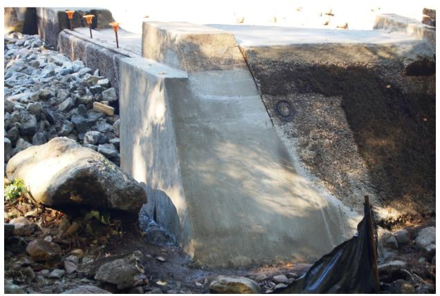
The picture below was from 1990 showing thea stump that the dam was poured around. 25 years later the stump is still there but deteriorating with additional organic growth (shown in the picture bottom right after it was cleaned out). This was repaired by removing the stump, installing pins to hold the whole structure together and pouring concrete into the void
