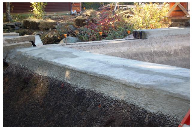
Cement on the top of the dam was pitted and flaking. This was repaired with a strong grout material as shown in these two pictures.
